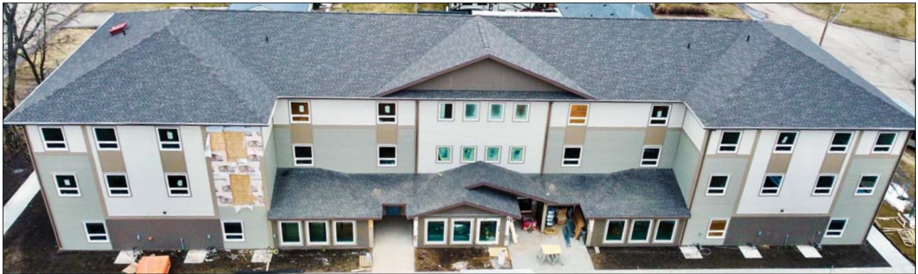
The Cobblestone House in Moosomin is planned to be open in June. Jim Yeaman of Care by Design spoke about plans for opening the long-term care and assisted living facility at the Chamber of Commerce meeting in Moosomin in April.
