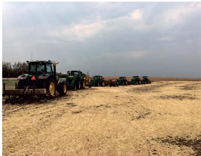
Pictured above is Enbridge laying down straw as part of earlier Line 3 right-of-way reclamation work in southern Saskatchewan.
